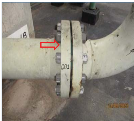
Picture 12 Flange Found in good condition
