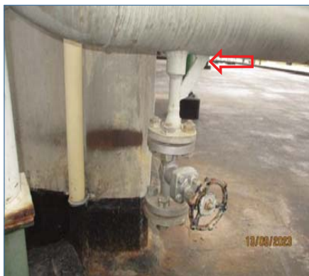
Picture 11 Small-bore and Gusset plate Found in good condition
