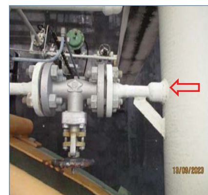
Picture 6 Small-bore and Gusset plate
